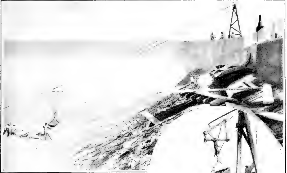
How the Stone and Old Concrete Were Removed from the Basin by the Improved Cableway
